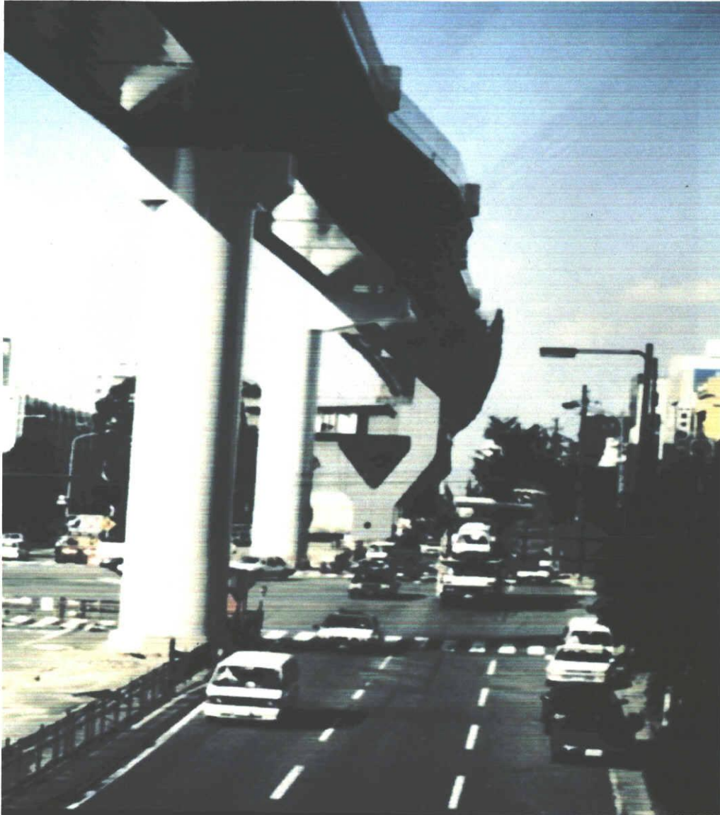
Fig.1-1 Elevated highway bridge pier used in the urban areas, Japan
