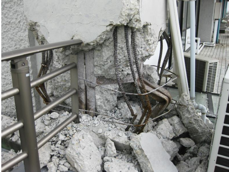
Figure 9: Base of boundary element at third floor
