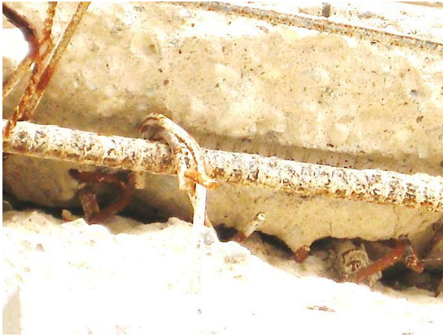
Figure 12: Close up of web-beam joint
