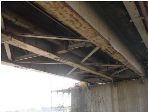
Photo 1.1 Corrosion of bridge and deterioration of protective coating
